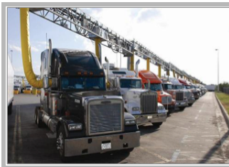
Grid or Solar Powered TSE: A/C, Power
