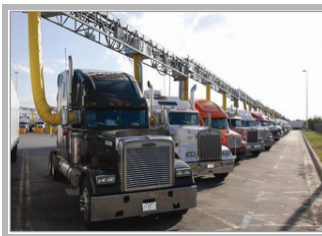
Grid or Solar Powered TSE: A/C, Power
